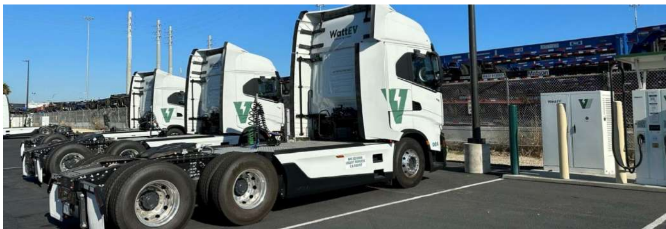
Figure 12 Trucks charging via Megawatt charging system (source: zerovatech.com)
