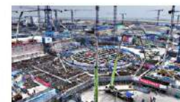
Construction of second Shidaowan Hualong One begins New Nuclear - Thursday, 8 May 2025
