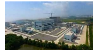
HTR-PM, China, 2x110 MWe HTGR in operation
