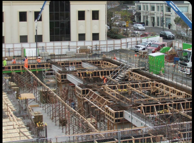
Stage 2 Rebuild foundations
