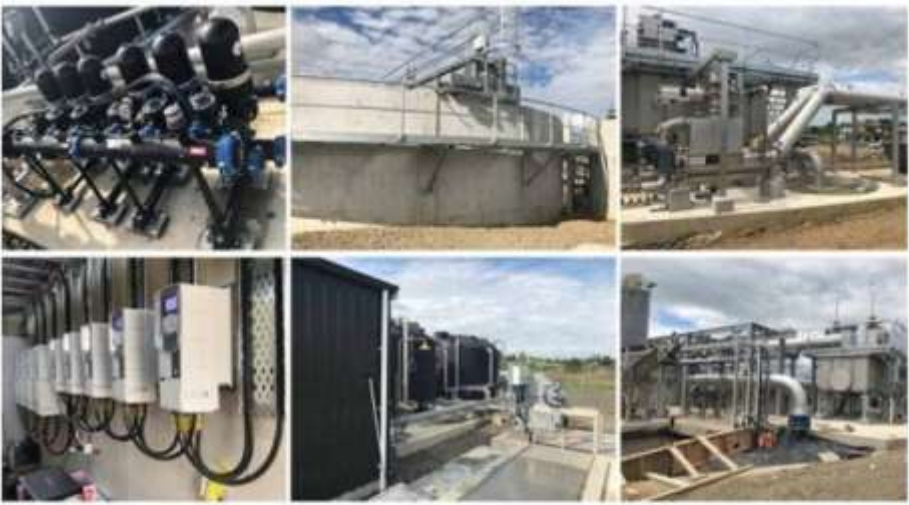
Finishing touches were recently put on the upgraded Te Awamutu Wastewater Treatment Plant while a new plant for Cambridge is in the planning stage
